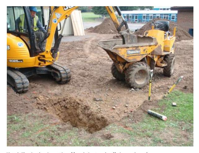
Plate 3. The site showing cutting of foundation trenches (facing north-east)
